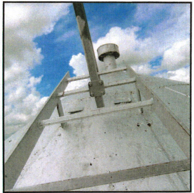
Shell/Roof ladder safety climb bracket properly fastened to ladder.
