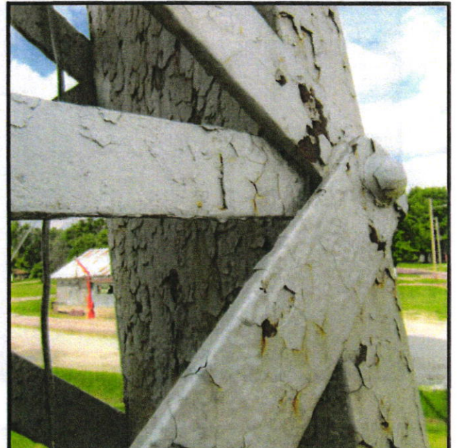
Cracking and peeling of several layers of paint.
