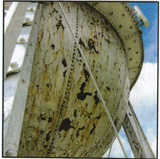
Tank belly coating failure.
