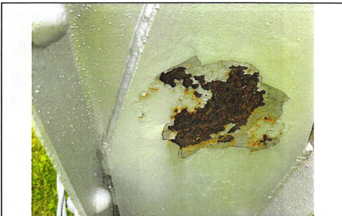
Photo 4: View looking at peeling paint on water tower base.
