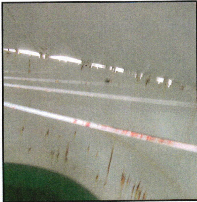
Coating failures. Eave gap opening. Spider rods.
