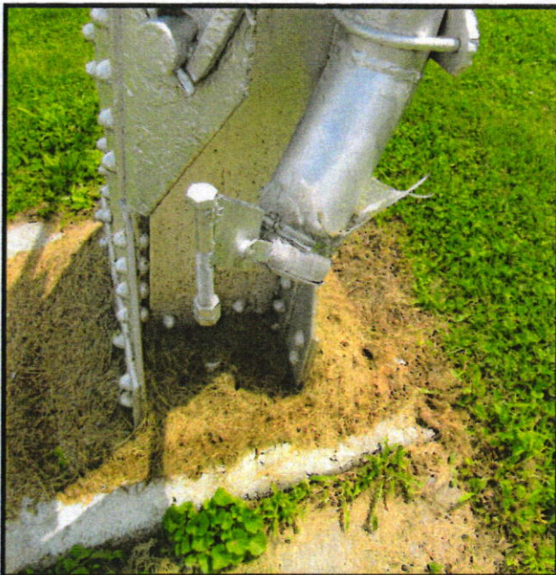
Overflow terminates above grade and has screen and flapper gate.
