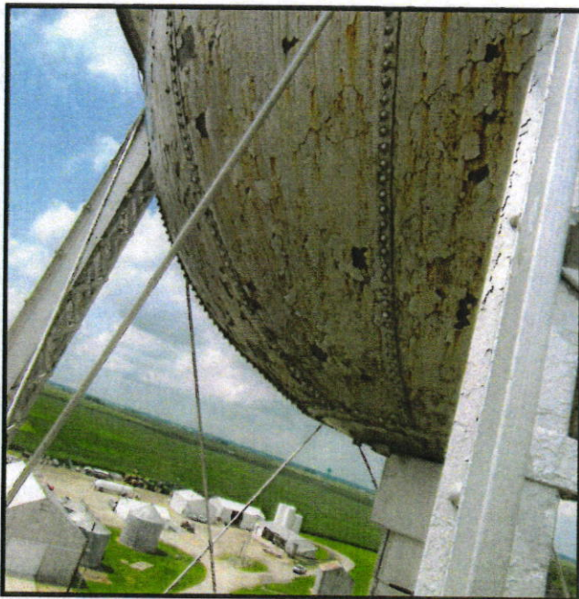
Tank belly coating failure.
