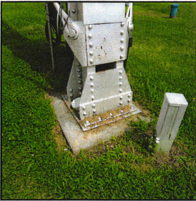
Foundation pads are in good condition above grade.
