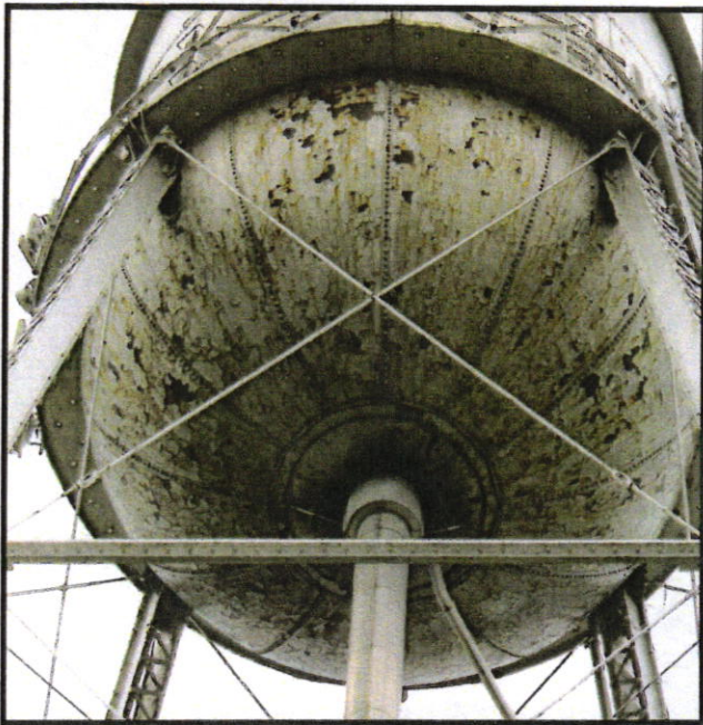
Exterior coatings in very poor condition and will require full removal prior to new coating system application.
