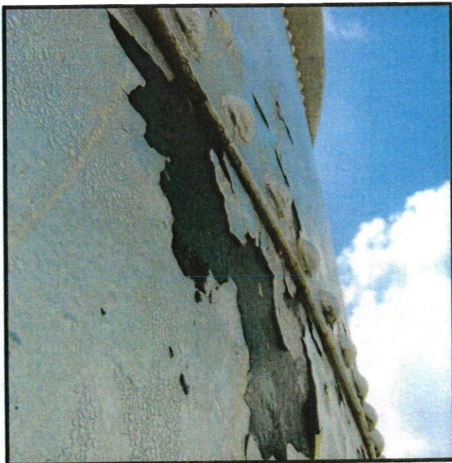
Coating failures on tank shell.
