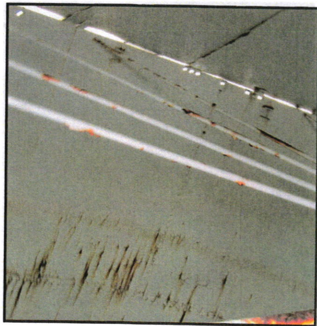
Tank interior wet coating failures.
