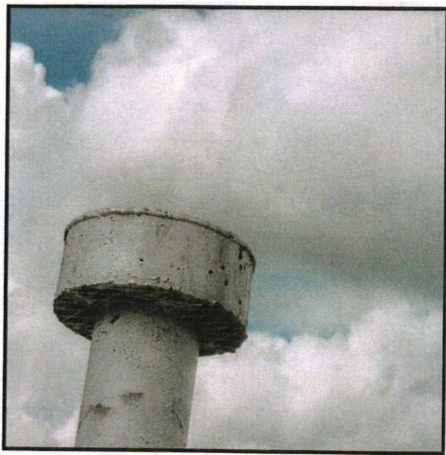
Roof vent does not meet current standard.
