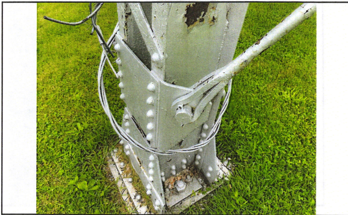
Photo 5: View looking at peeling paint on water tower base.
