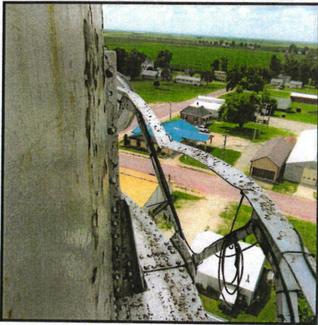
Balcony top rail damaged and bent in towards tank shell.
