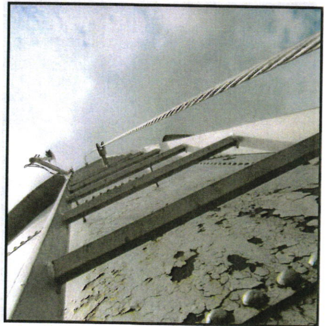
Shell ladder equipped with cable safety climb.
