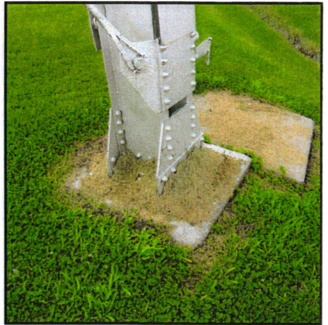
Foundation pads are in good condition above grade.
