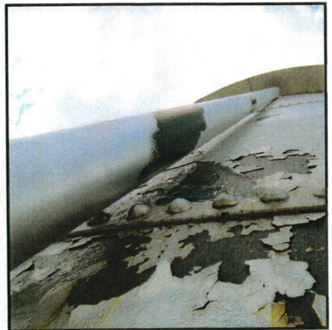
Coating failures on tank shell.
