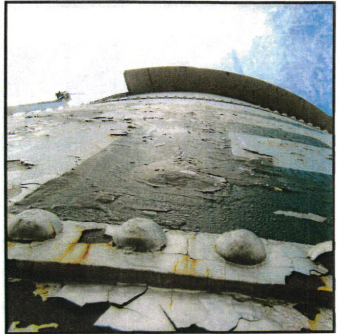
Coating failures on tank shell.
